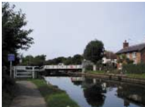
The bridge at Hall Lane
